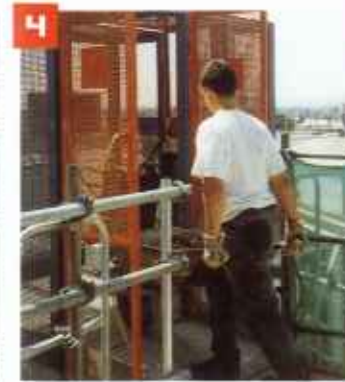
4 The landing levels are secured by 1.1 m high galvanized safety gates. These come complete with cable for serial connection and integrated control.
