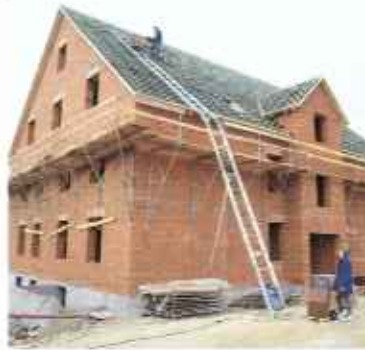
Inclined lifts with steel wire rope
