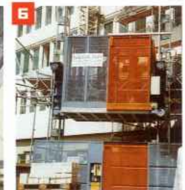
6 When the cage moves into the ground station, the cage door at the front is unlocked automatically and can be opened together with the sliding door of the ground station.
