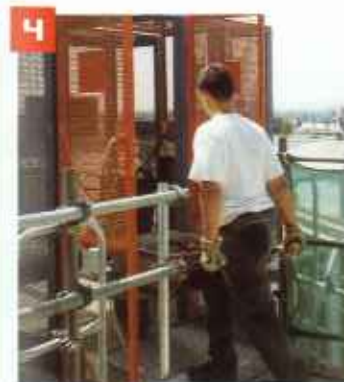
4 The landing levels are secured by 1.1 m high galvanised safety gates. These come complete with cable for serial connection and integrated control.
