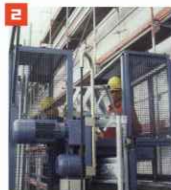
2 Easy and rapid assembly from inside the hoist cage: open assembly tunnel, put on mast section, raise mast, tighten the captive screws (M16) with self-locking nuts – ready.
