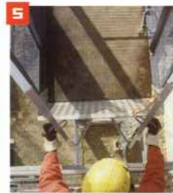
5 As soon as the cage reaches the landing level, the cage door is unlocked automatically. When it is opened, a gangway with lateral protection unfolds automatically for safe passing to the building/scaffold.
