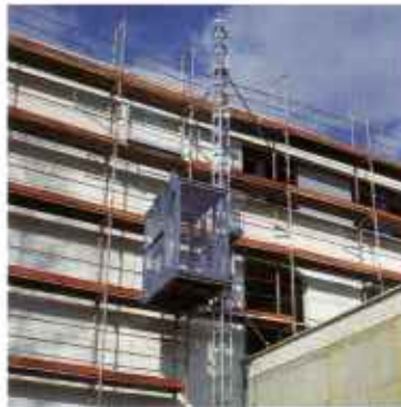
Passenger/material hoists
