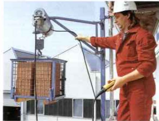
GEDA swivel arm hoists can help save a lot of time and energy on site: Ball bearing hooks and pulley block act as twist preventer.
